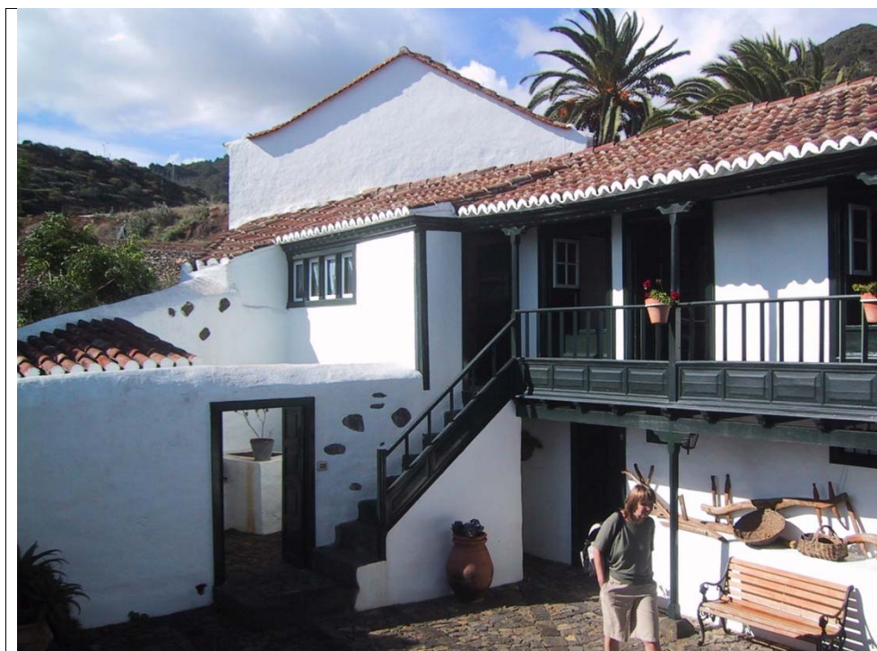
12.4 – Vista general del patio interior
