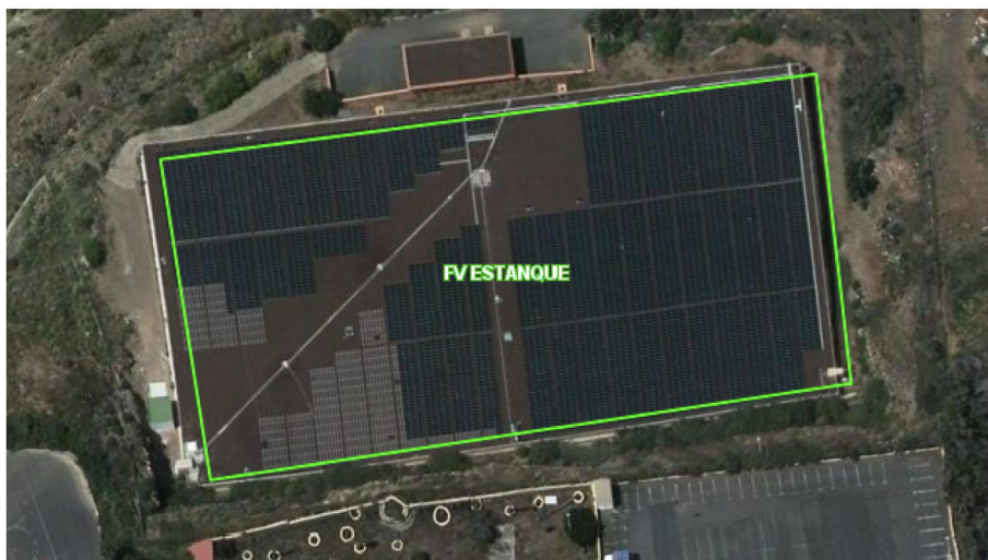
Fig. 7. Uncovered water deposit with a photovoltaic installation in Arinaga (Gran Canaria).
