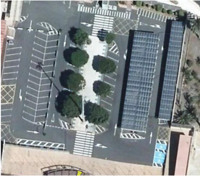
Fig. 6. Photovoltaic parking space in INFECAR (Gran Canaria).
