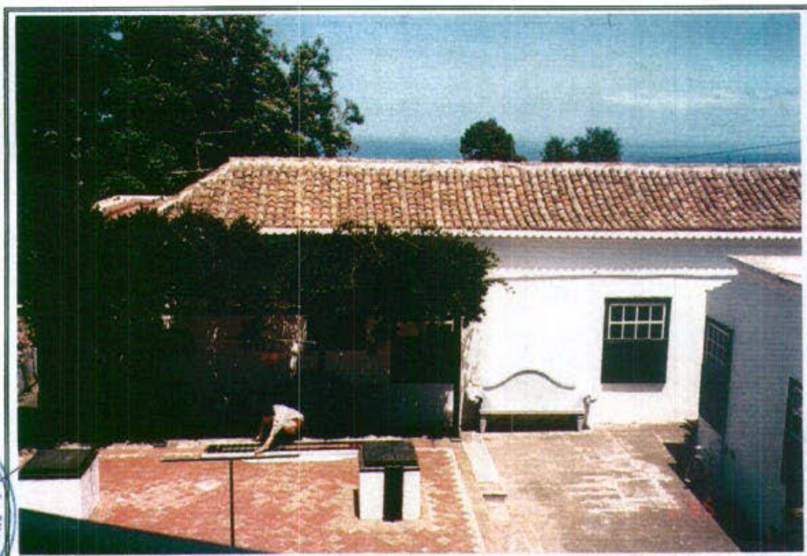
50.3 - Vista general patio interior
